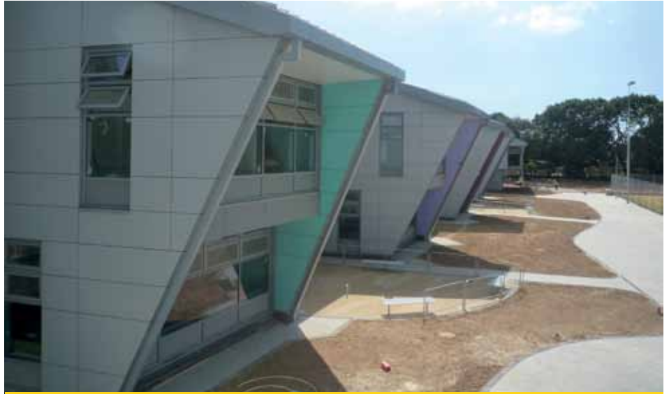
Bexhill High School - Work in progress
