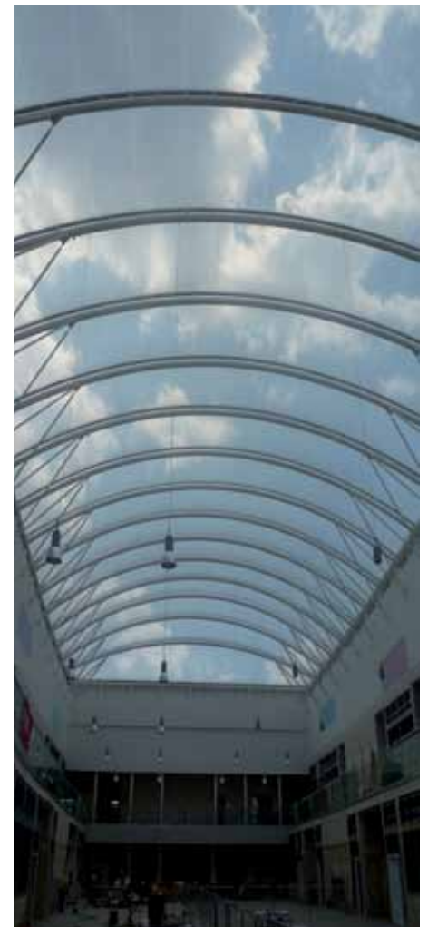
Bexhill High School - ETFE air filled roof
